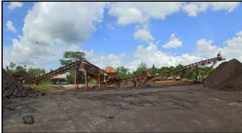
Gambar 1. Rangkaian Crushing plant double roll crusher
